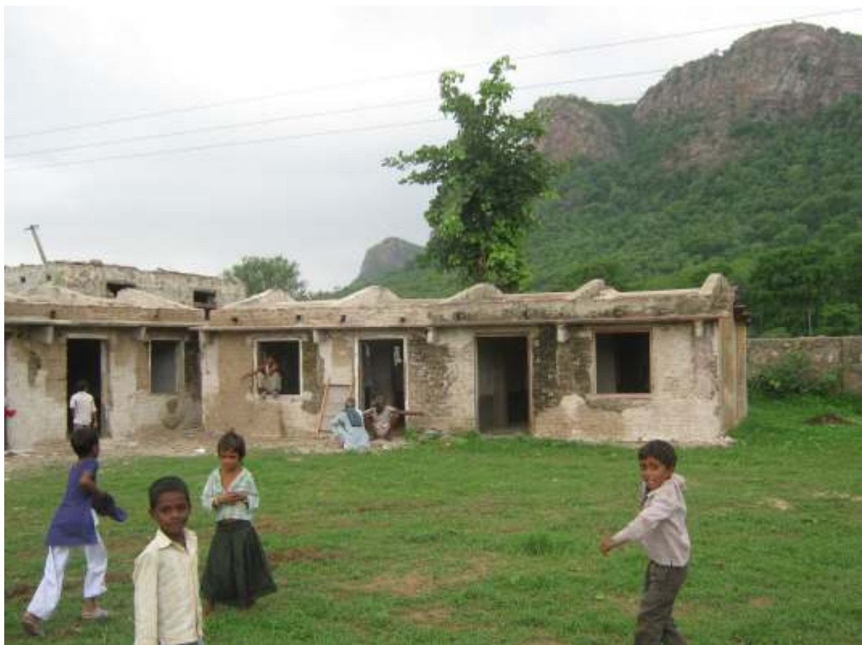
The new school campus for Uday Samudayik Pathshala Bodal
