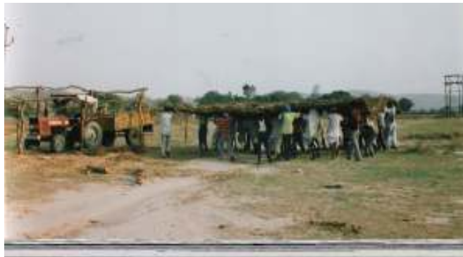
School under construction
